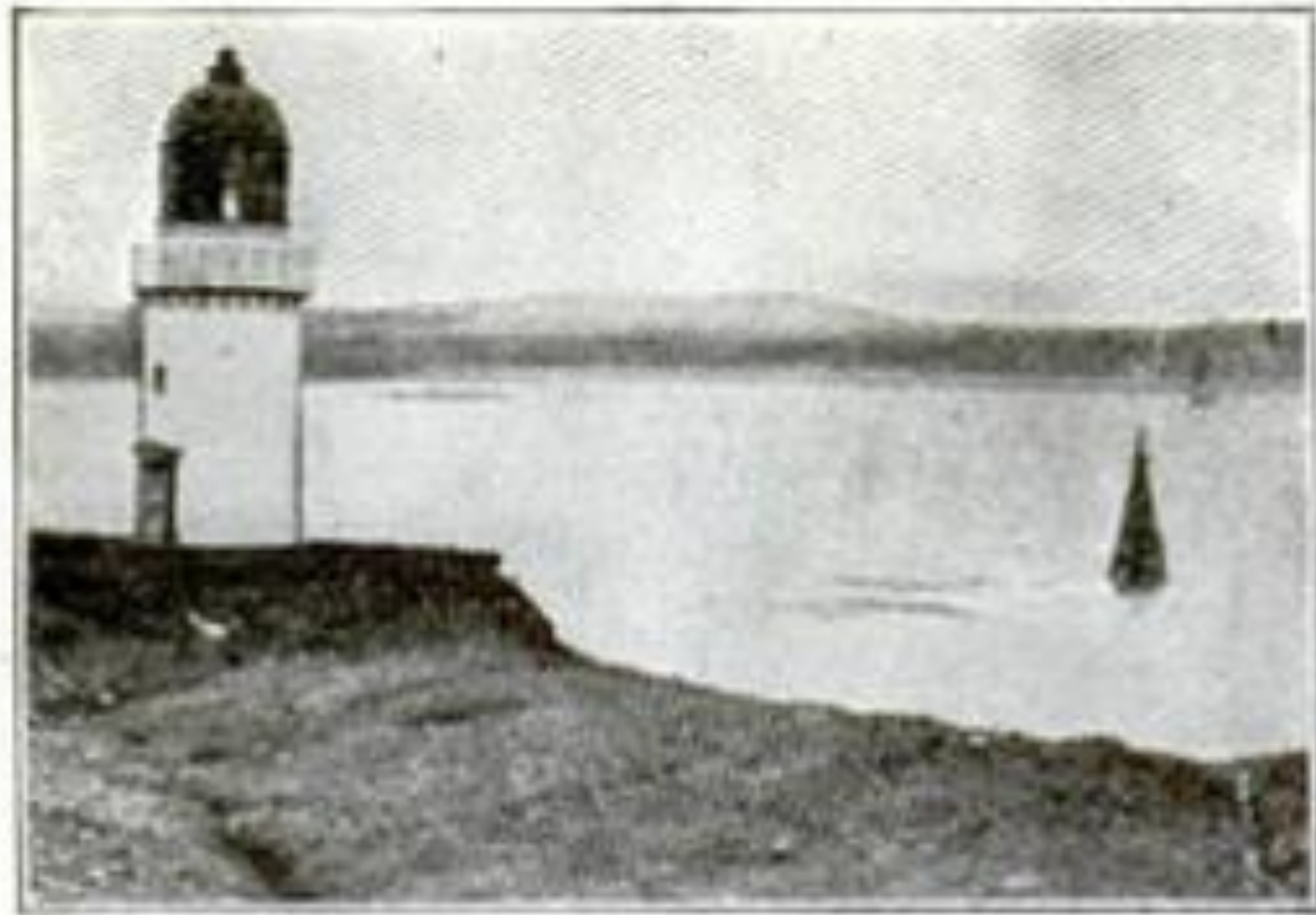
A LAMPLESS LIGHTHOUSE —This strange but ingenious beacon is located at Arnish Rock, Stornoway Bay, in the Hebrides, Scotland. It is a cone of cast iron plates, surmounted by an arrangement of prisms and a mirror, which reflect the light from the lighthouse on Lewis Island, 500 ft. distant across the channel.
